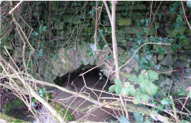
Culvert in F11
