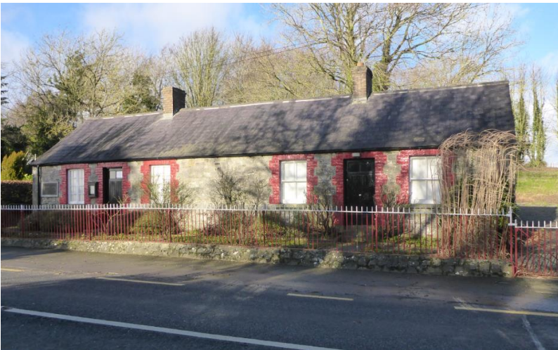
Ledwidge Museum cottage on N51, facing N
