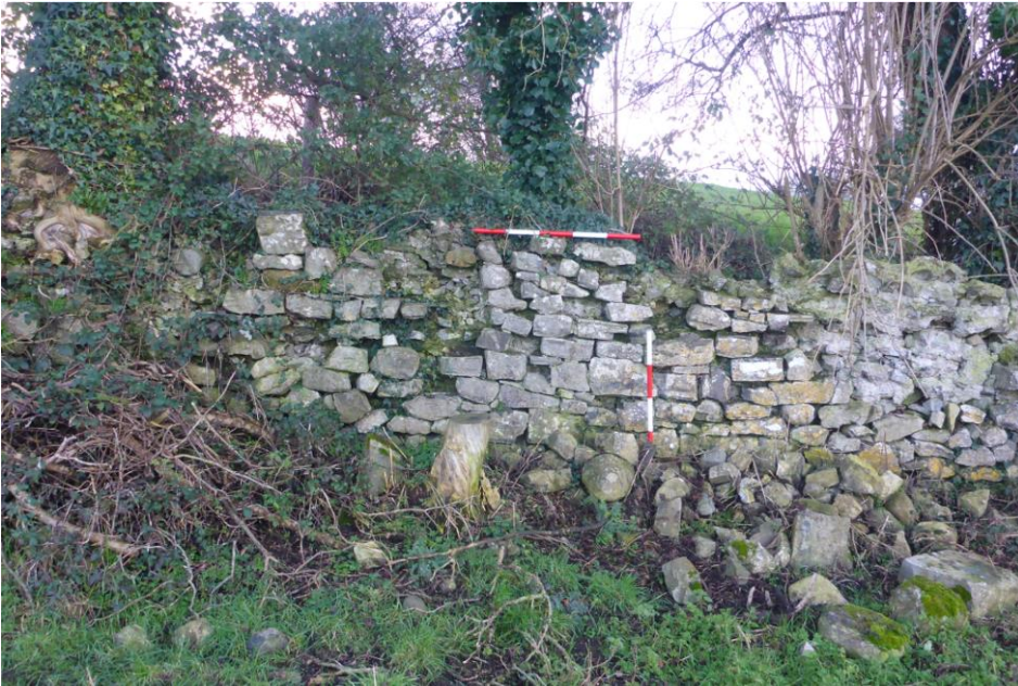
Retaining stone field boundary wall between F11 and F12
